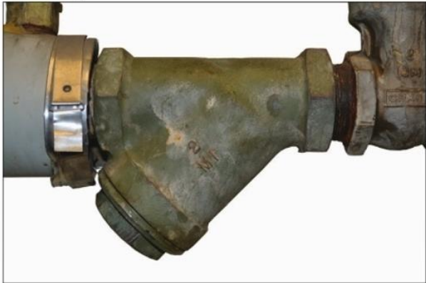
Figure 9: Y pattern strainer
